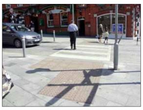
Figure 4.24: Example form Drogheda, Co. Louth, of red tactile paving at a zebra crossing which has been toned down to balance the degree of contrast with higher specification materials.
