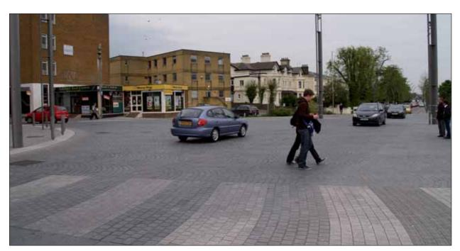
Figure 4.49: Shared surface junction in Ashford, Kent, UK, carries significant amounts of traffic and challenged conventions regarding traffic volumes along shared surfaces. An informal zebra crossing has also been marked adjacent to the junction to provide a place for less confident pedestrians to cross.
