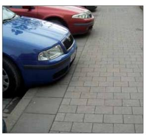
Figure 4.36: An example where a narrow verge is provided to ensure that vehicle overhangs do not intrude on the footway.
