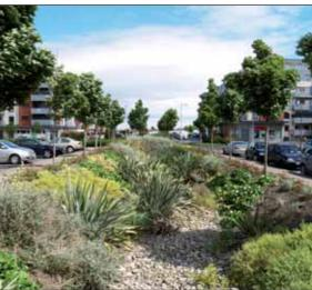
Figure 4.29: Examples of Sustainable Urban Drainage incorporated into a street in the form of a small 'swale' (top) and larger linear basin (bottom). These treatments not only assist in containing urban surface water run-off but also contribute to the sense of place by adding a unique feature.
