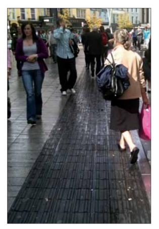
Figure 4.50: Examples from Cork city of the use of tactile paving that assist the visually impaired by guiding movement across a shared space.
