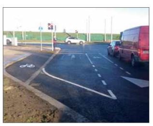
Figure 4.59: Left turning slips (left) generally offer little benefit in terms of junction capacity and increase the number of crossings pedestrians must navigate. They also allow vehicles to take corners at higher speeds, exposing pedestrians and cyclists to greater danger. Where a large number of turning movements occur, left turning lanes (right) with tighter corner radii should be used.
