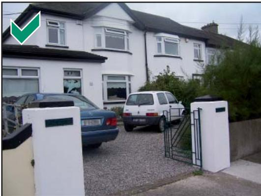
Permeable gravel on parking areas will allow natural drainage to occur
