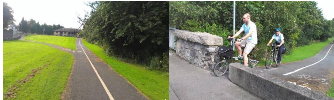
Steep incline to Dundrum Road and low wall restricting access
