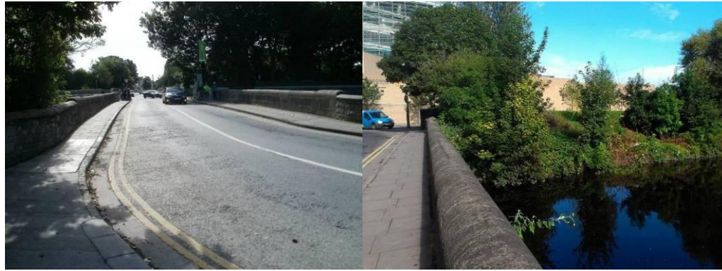
Lansdowne Road Bridge
