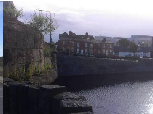
Upstream side of Bridge
