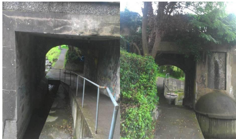
Classon's Bridge (North-East)
