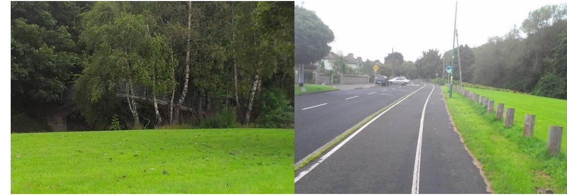
Existing Bridge to Lower Dodder Rd
