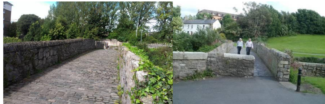
Old Bridge at Milltown
