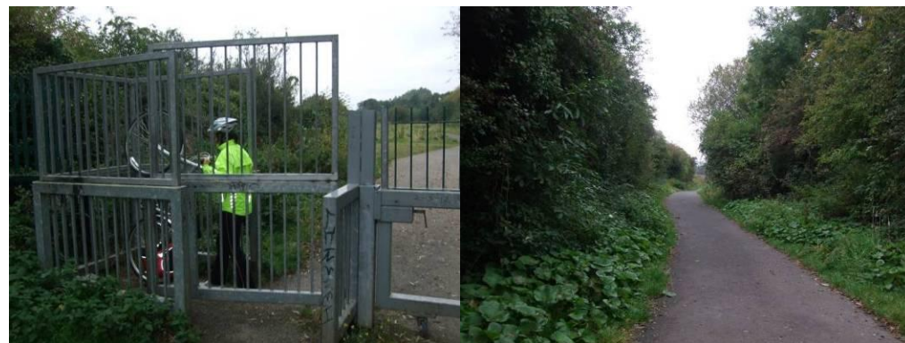
Pedestrian gate in Dodder Valley Park Overgrown vegetation along the route
