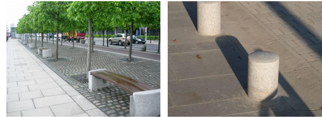
Seating used as bollards to separate corridors and low key discrete bollards - Dublin Docklands
