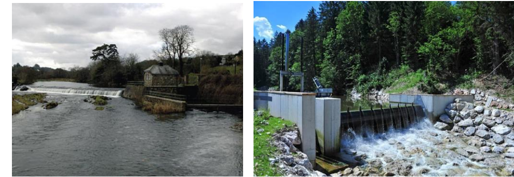
Small hydro-electric power stations on the Bandon River in Cork and in Austria
