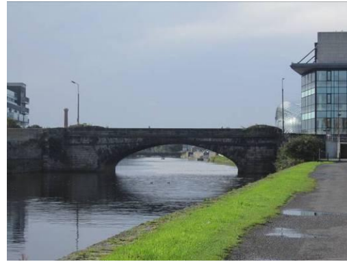
Ringsend Road Bridge
