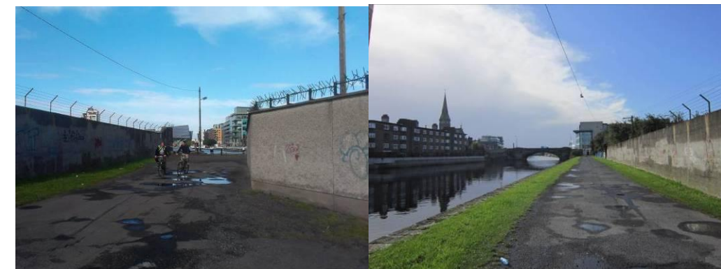
Route from Lock
