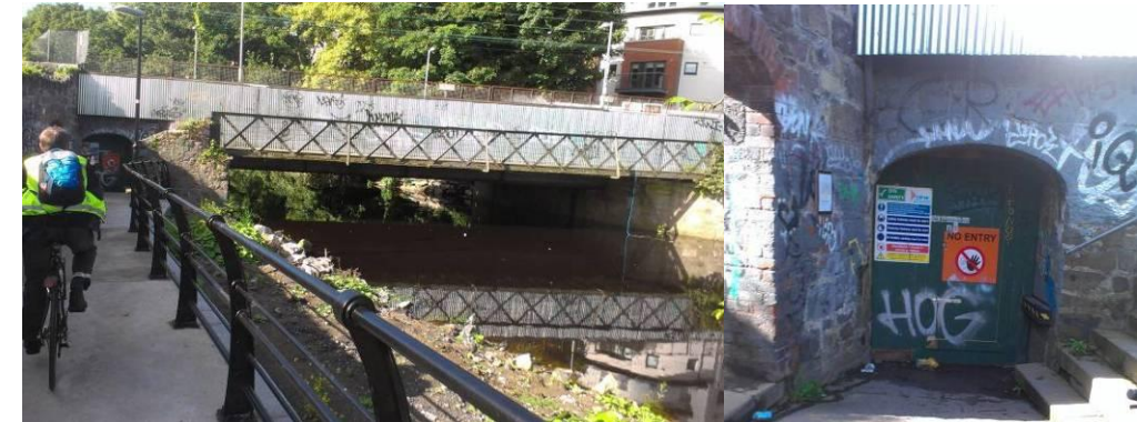
Railway Bridge Across Dodder
