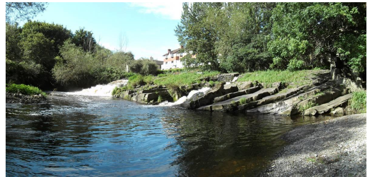
Beech Hill Weir looking from northwest side of river
