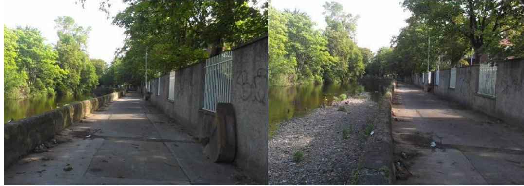
Railway Crossing to Beatty's Avenue
