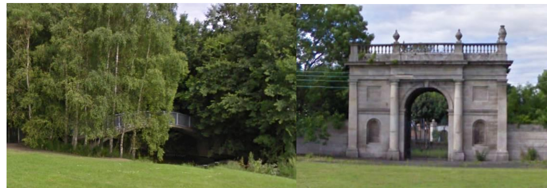
Existing Bridge at Lower Dodder Road
