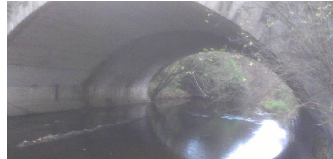
Arch Bridge over Dodder at Rathfarnham Road
