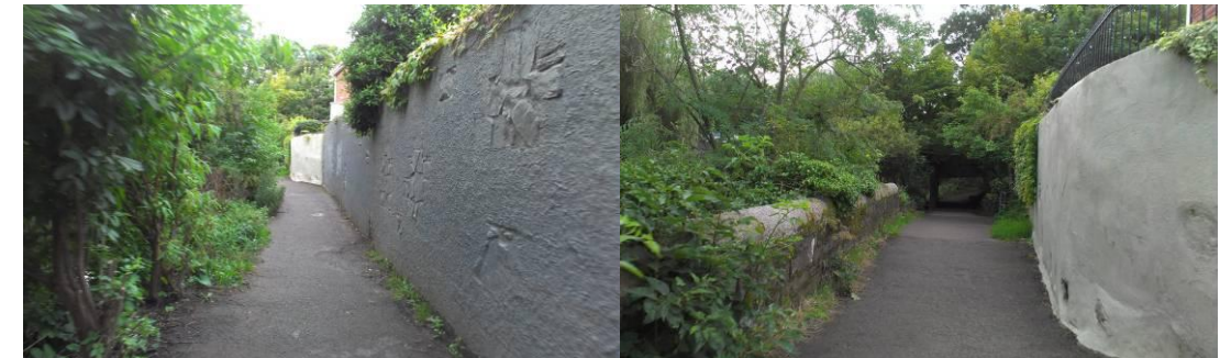
Approach to Orwell Road Underbridge
