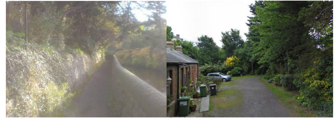
Middle Section with Retaining Walls
