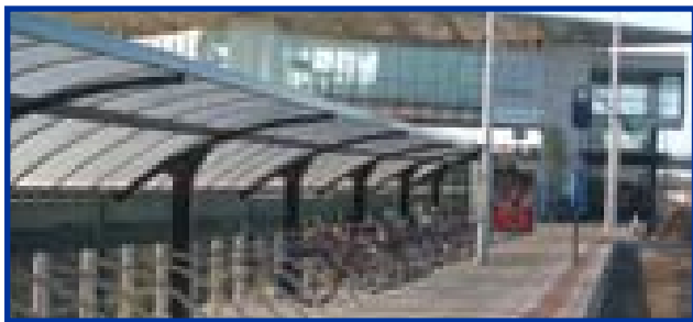
Cycle facilities provided adjacent to new Adamstown railway station
