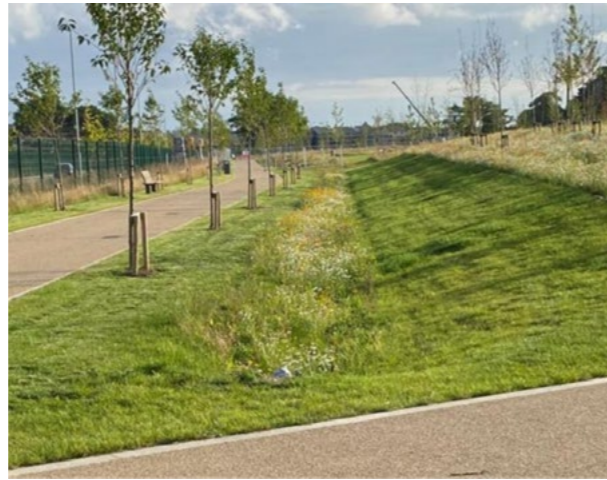
Image shows swale (linear basin) with potential for storing rainfall runoff (Tandys Lane Park, Adamstown)
