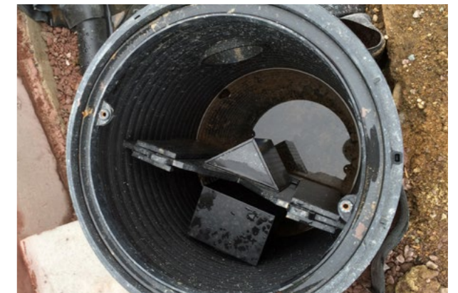
Images show a protected orifice plate within shallow chamber and weir made from recycled plastic planks.
