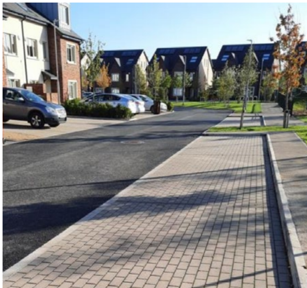
Image shows permeable paved on street carparking - Cuil Duin, Cooldown Commons
