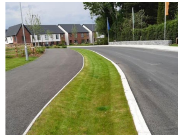
Image shows Collection of 'sheetflow' rainfall runoff over flush kerb into a shallow swale. Strategic Housing Development, Newcastle, Co.Dublin
