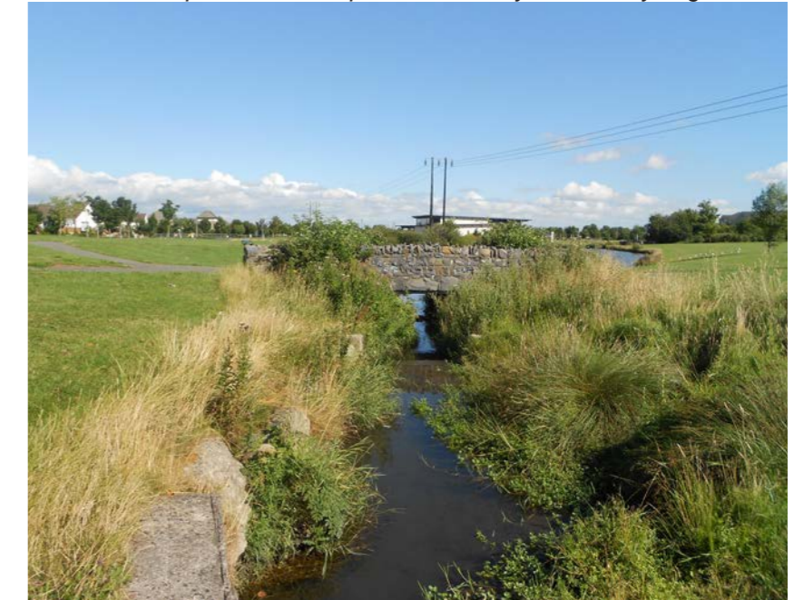
Utilisation of Open Stream as part of SUDS System - Ballycragh Pk.
