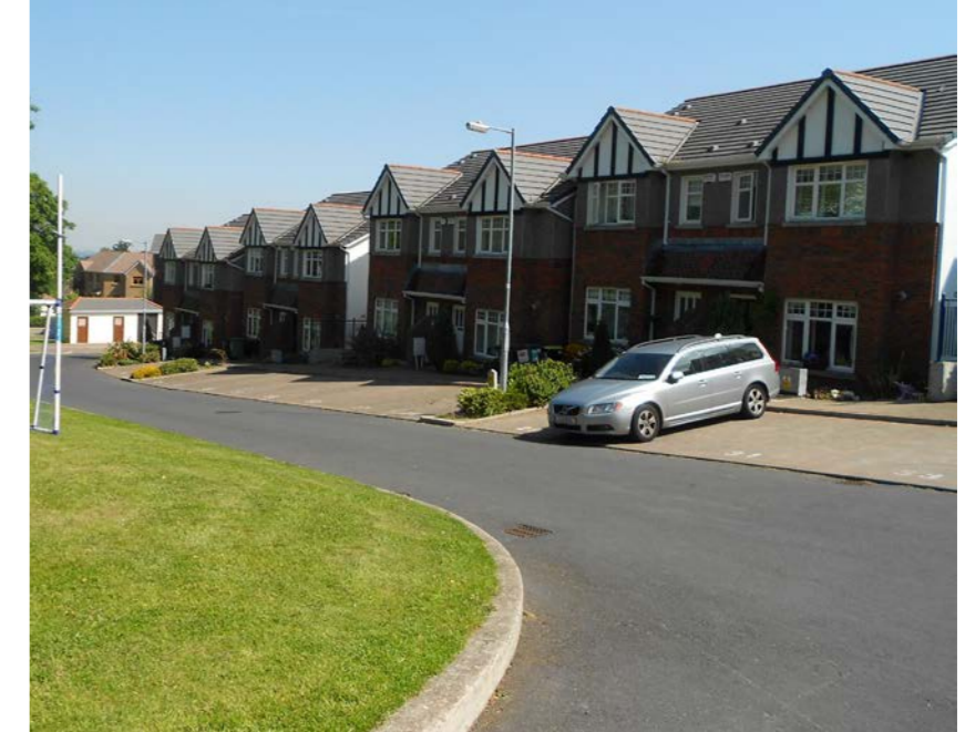
Photo 2.3 Semi-Detached Housing in Stocking Wood
