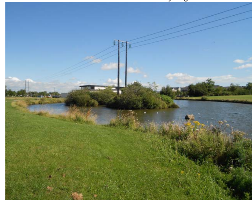
SUDS Attenuation Pond within Parkland - Ballycragh Park
