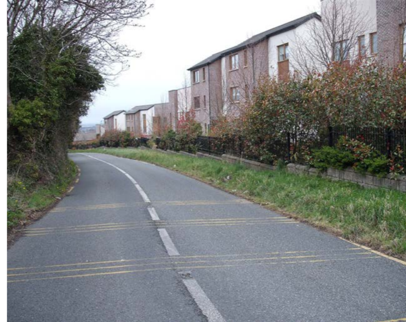
Photo 2.2 Urban Style Housing in Hunterswood adjacent to Gunny Hill
