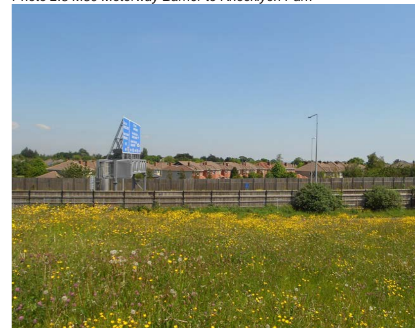
Photo 2.8 M50 Motorway Barrier to Knocklyon Park
