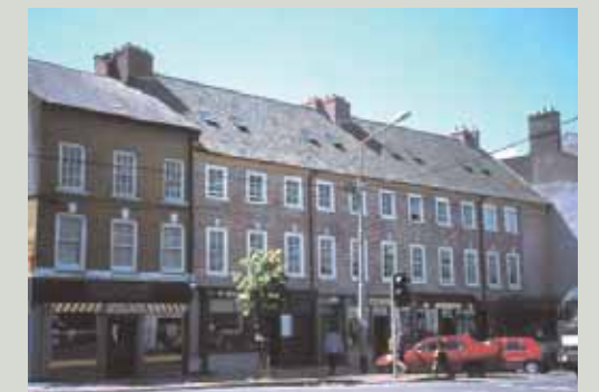
This restored terrace of early eighteenth-century houses retains the original appearance of the fully visible sash frames, which is quite different to the later house on the left
