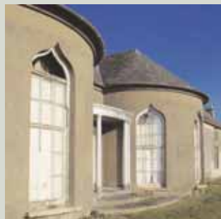
Although this house has been left disused and the windows vandalised, it should not be presumed that what remains cannot be repaired. Each window should be assessed and tailored repair schedules made up for each. If it is found that the parts of a window are beyond repair, accurate profiles should be drawn up for the fabrication of new sashes or frames, and the historic glass should be salvaged for use in the new work
