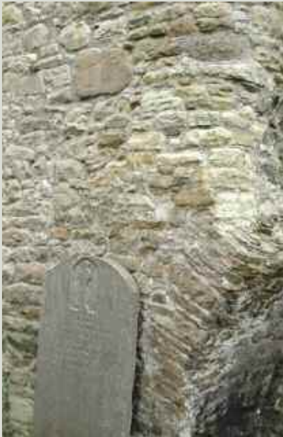
Sandstone rubble in a masonry wall
