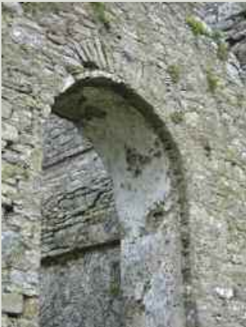
Even buildings which have stood as ruins for centuries can retain traces of internal plaster. These are most often found in sheltered parts of the building such as here on the intrados of an archway
