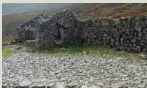
Surviving granite paving to an external yard in a ruined mining village
