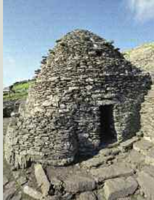
The early mediaeval monastery of Skellig Michael, off the coast of County Kerry included a series of beehive-shaped cells of drystone construction built to withstand the harsh climate at the edge of the Atlantic ocean. Circular in shape from the outside, the internal spaces of the cells are in fact square or oblong
