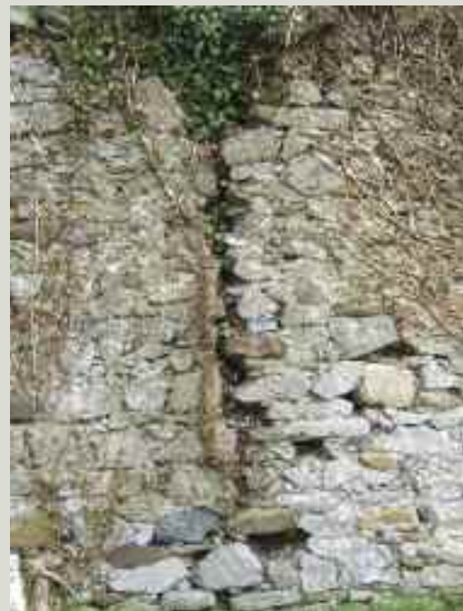
Vertical cracks can be more common in walls where few long facing stones were used. Longer stones create a stronger bond than smaller stones
