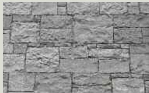
Snecked masonry, sometimes called random ashlar, was built in discontinuous courses with small stones or snecks introduced to break courses. The stones required cutting but offered economy in material as smaller stones could be used. This style of construction was first used in the nineteenth century and is distinctly Victorian
