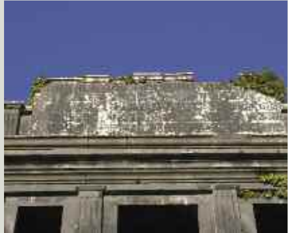
Limestone ashlar in a masonry wall
