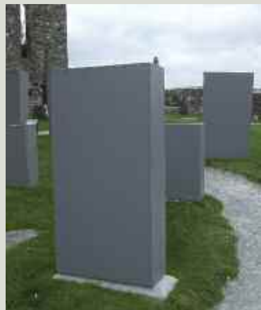
Graveyard with headstones protected by plywood casings in advance of conservation works to the adjacent structure
