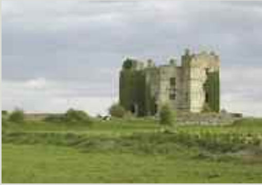
At Loughmoe Court, County Tipperary, the original fifteenth century tower house (seen on the left) was extended in the first decades of the seventeenth century with the addition of a semi-fortified Jacobean mansion
