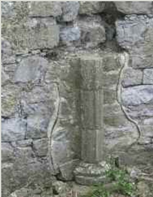
A method of distinguishing between old and new masonry in repair work was used by the Office of Public Works in the mid-twentieth century and can still be seen on many national monuments today. The technique involved separating the new from the original by the insertion of a strip of felt. This technique is no longer used today
