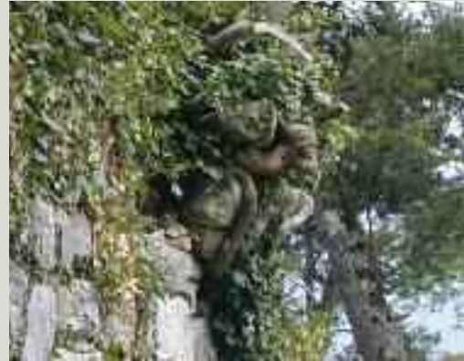
Ivy will displace stones as its stems thicken and can become part of the structure, holding up the stones it has dislodged
