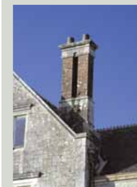
Chimney stacks are difficult to maintain as they are often the least accessible parts of the building but they are also the most exposed. Their condition can usually be monitored from ground level using binoculars
