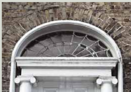
The cleaning and repair of fanlights is a delicate task which should be left to a specialist
