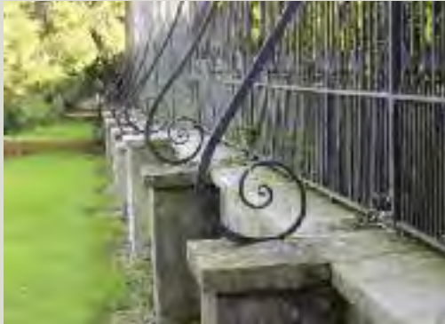
Tapering scrolls are another common feature of wrought ironwork
