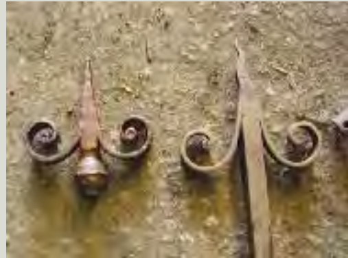
While modern welding techniques are not ideally suited to traditional ironwork, a skilled craftsman may be able to apply modern welding to repairs to a level that is visually acceptable. The finial on the left has been forge welded and hammered down to a point, while the finial on the right has been electric arc welded and then hammered into a point in the traditional way
