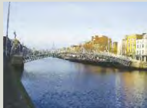
Dating to 1816, the Ha'penny Bridge is the oldest cast iron bridge in Ireland. It is also one of the earliest cast iron bridges ever made. Its parts were fabricated by the famous English firm Coalbrookdale, also responsible for making the first cast iron bridge in the world, which still stands at Ironbridge, Shropshire, England
