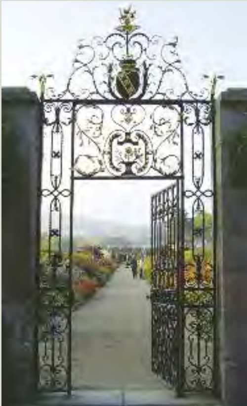
Delicate leaf-work is typical of wrought ironwork
