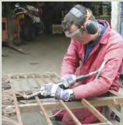
A needle gun can be effective at removing corrosion material, but can be damaging to the surface of ironwork if applied with too much pressure (Image courtesy of Historic Scotland)
