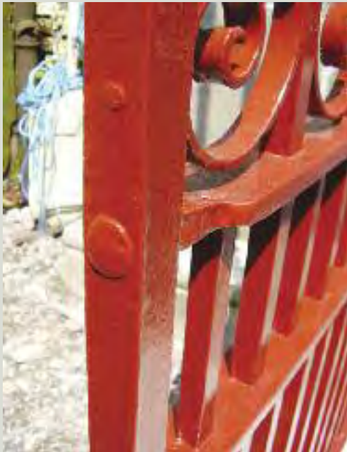
Wrought iron was traditionally assembled by means such as forge welding, collars, scarf joints, and mortice-and-tenon joints
