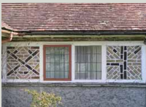
The Arts and Crafts Movement in the late nineteenth century promoted the use of handcrafted building materials, including handmade bricks, as in this example of a house at Talbot's Inch village, Co. Kilkenny designed by the architect William A. Scott and built 1896-1904
