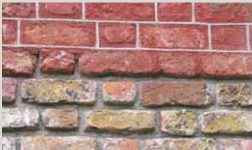
Tuck pointing in practice
