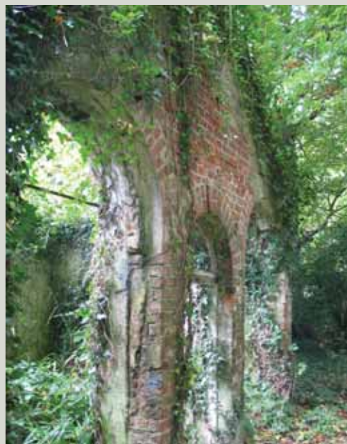
Ruined garden house of brick at Newbridge House Demesne, Co. Dublin
