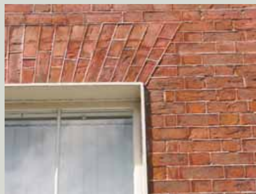
A typical Irish eighteenth-century flat arch window head. It differs from similar English flat arches of the period in that the arch does not splay widely at either end
