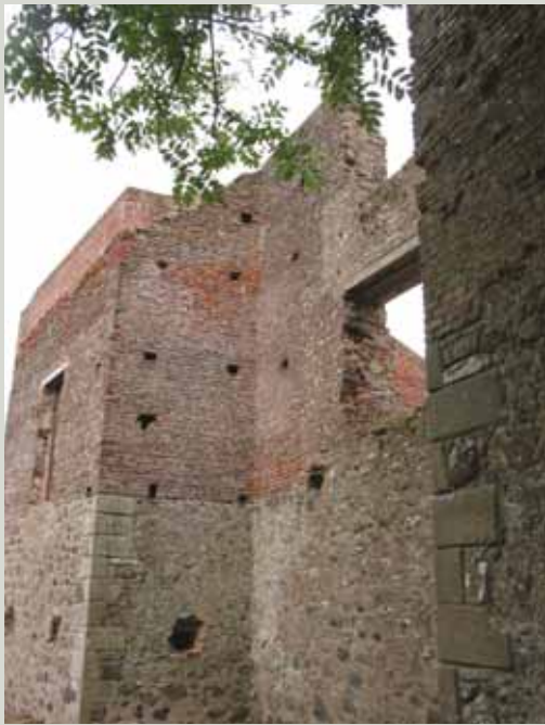
Mountjoy Fort, Co. Tyrone, built c. 1603, is the earliest known surviving Irish building where brick was used as the substantive building material for walls
