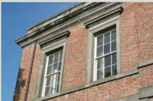
The brick façade, with stone dressings, of Cashel Palace, Co. Tipperary, was designed by Edward Lovett Pearce before 1729 for Archbishop Goodwin
