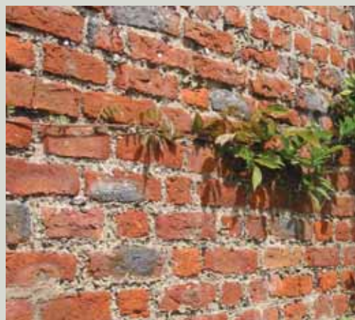
Garden walls lined with brick at Beaulieu House, Co. Louth. The orientation of garden walls was the subject of several gardening manuals in the early eighteenth century. The recommendations were that walls should face south-east, south-west, north-east and north-west. The first two, for example, were considered good for best fruit; the latter for plums, cherries and baking pears
