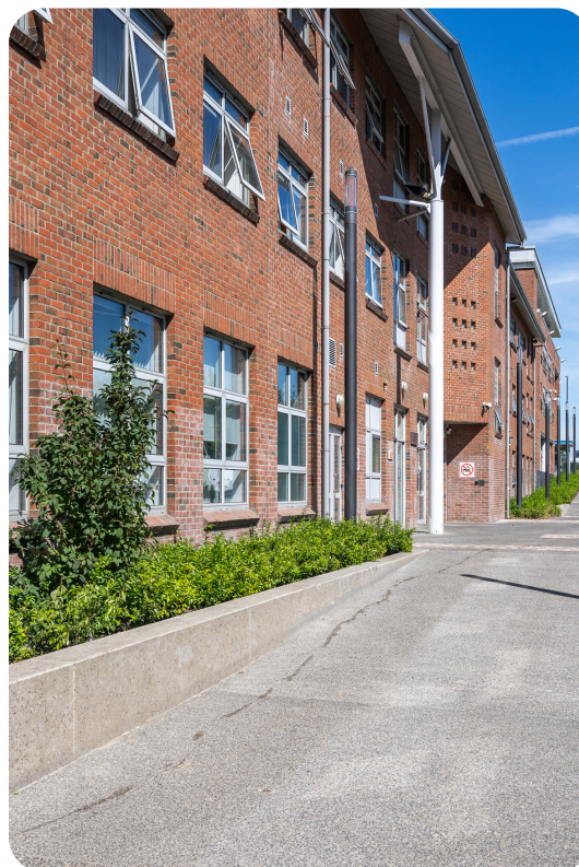
Side entrance to County Hall building, beside car park
