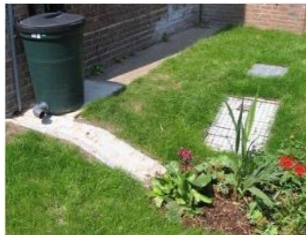
Images: downpipe is directed through water butt and then onwards to the raingarden .
