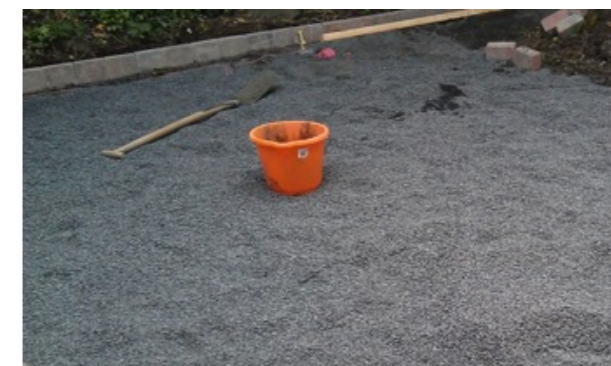
Images: stages of construction
