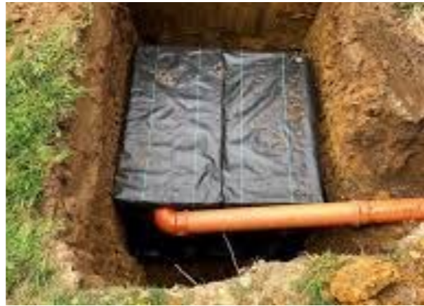
Image: soakaway being installed
