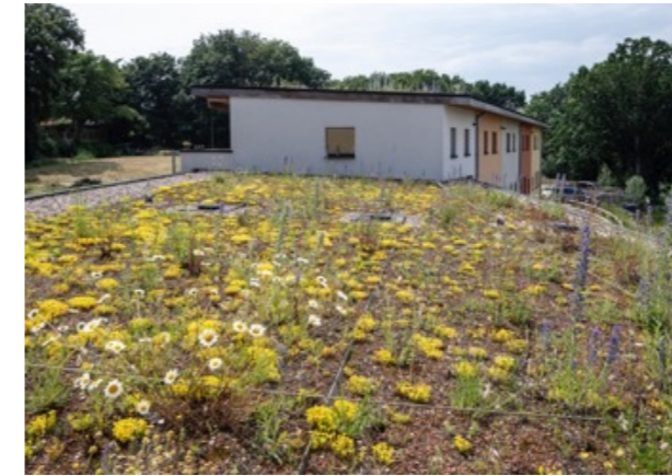
Image: green roof installed on a gently sloping roof
