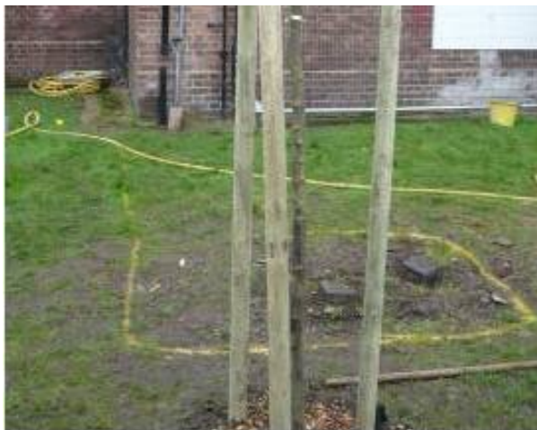
Image: recently planted tree and rain garden redesigned around the underground services
