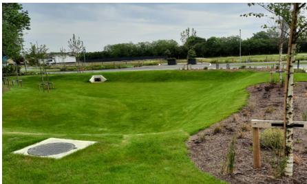
a Green Roof, a natural planted surface replacing the traditional roof that can absorb rainwater. A grassed Swale, or ground depression, slows the flow of surface water from the car park.
