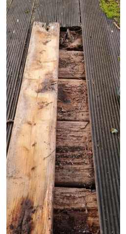
Bridge Deck is rotten
