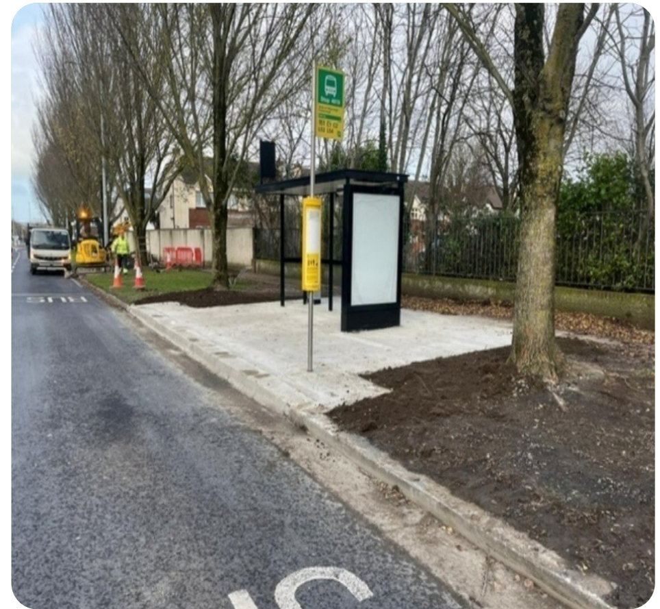
Fig 3.4 New Bus Shelter at Foxborough, Balgaddy Rd
