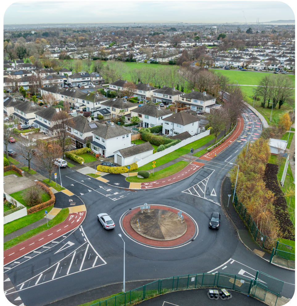
Fig 1.1 Ballycullen Drive - Avenue Junction, Firhouse
