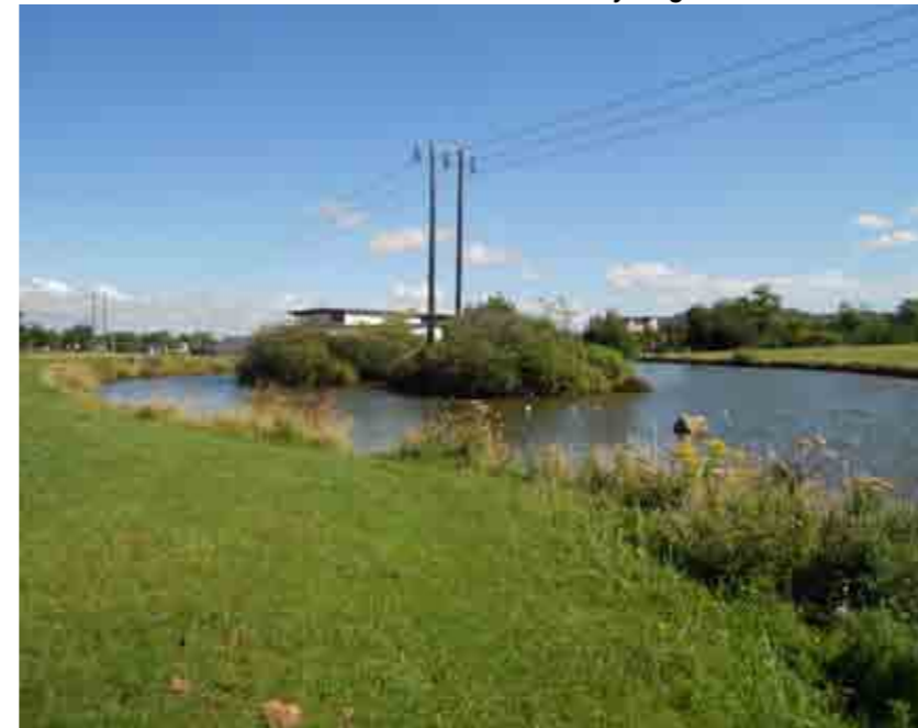
SUDS Attenuation Pond within Parkland - Ballycragh Park
