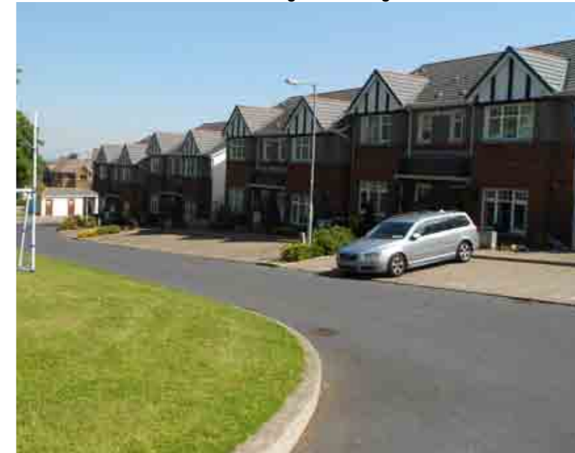
Photo 2.3 Semi-Detached Housing in Stocking Wood
