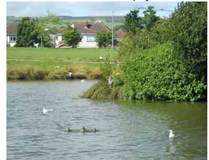
Island Habitat within Local SUDS Pond - Ballycragh Park
