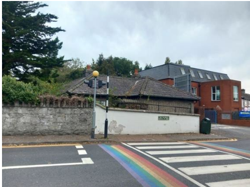
RPS. 153 Convent Road, Clondalkin Detached Multiple Bay Single Storey Former Gate Lodge.
