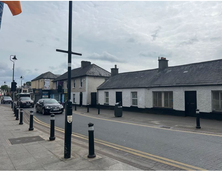
Plate 2 The southern side of main streets is characterised by a stepped roof profile and vernacular building forms with hipped pitched roofs and vertical emphasis on the upper floor windows.
