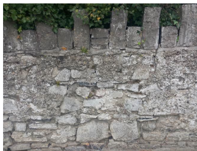
Plate 4 Early limestone wall on Tower Road, with weathered roughcast render and 'cock and hen' capping stones.
