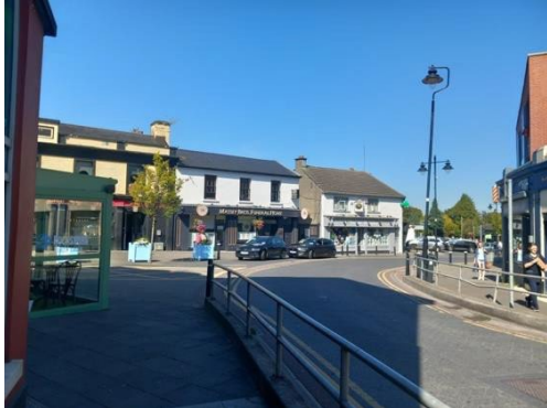
RPS. 143 Patrick Massey, Funeral Home, Orchard Lane, Clondalkin Semi Detached Three Bay Two Storey Building
