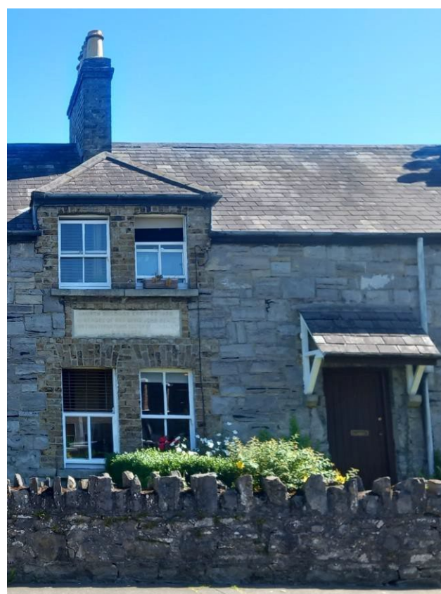
Plate 5 St. John's Cottages have exposed limestone walls, with buff brick quoins to the openings.
