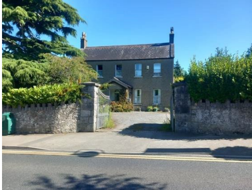
RPS. 419 Towerville, Tower Road, Clondalkin Detached, five bay, two storey house, c.1850
