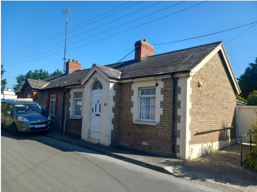
Plate 2 Typical cottage: buff brick with projecting gabled porch and pitched roof with red brick chimneys.
