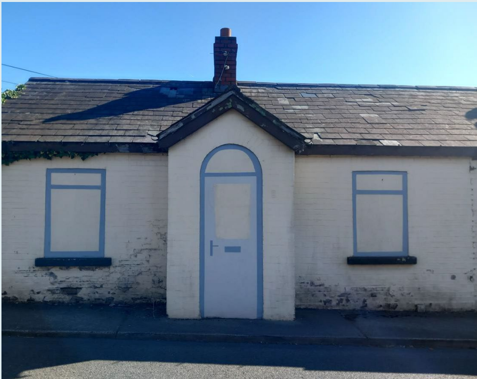
Typical dwelling house in St. Brigid's Cottages ACA
