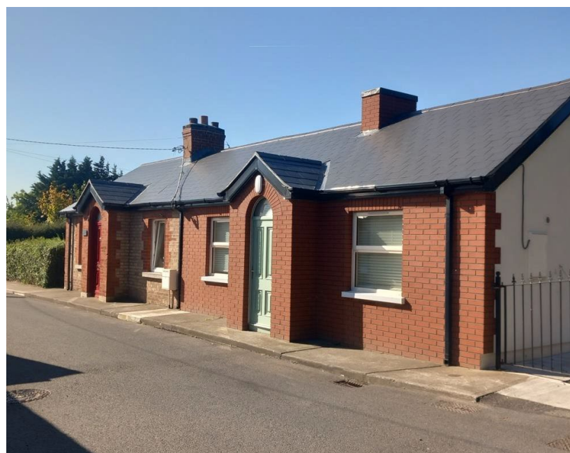
Plate 4 External alterations: External wall insulation has been applied to the structure on the right resulting in the loss of the original brick, the loss of the decorative brick quoin to openings, the loss of the granite stonework at the entrance, loss of the chimney profile and has introducing a stepped profile at the junction with the adjoining house.
