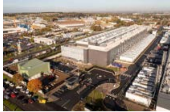
'Heat Works' Tallaght District Heating Network.
