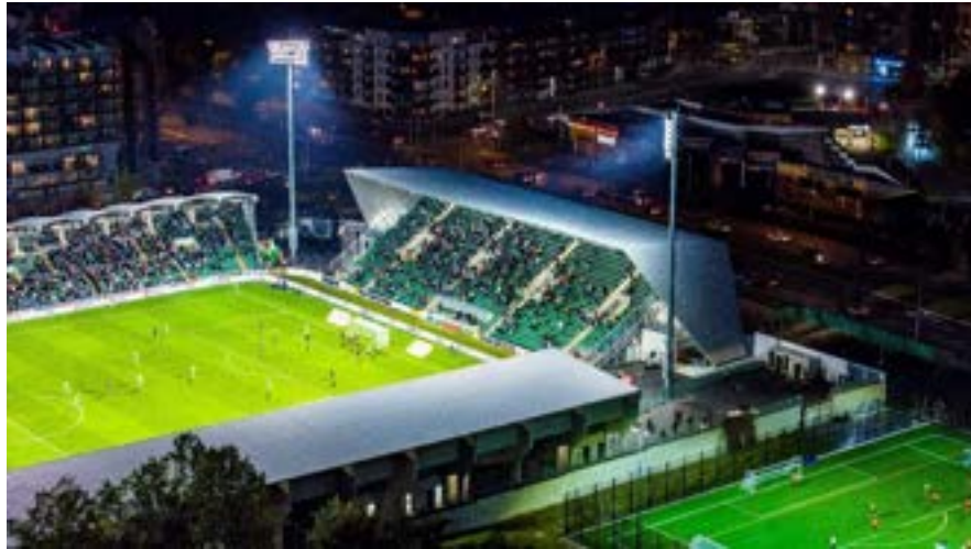
The Completed Tallaght Stadium 4 th Stand, now open, with the completed and open Sean Walshe Park Astro Turf facility in the right foreground
