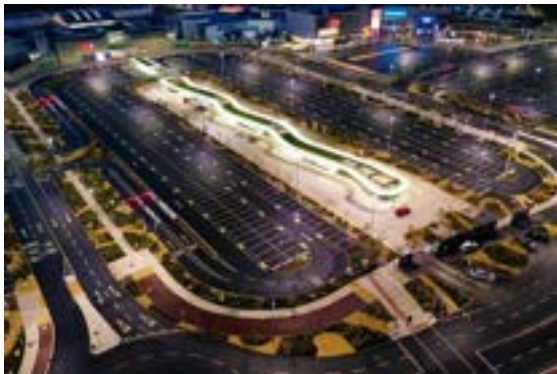
New BusConnects Plaza located at Liffey Valley Shopping Centre.
