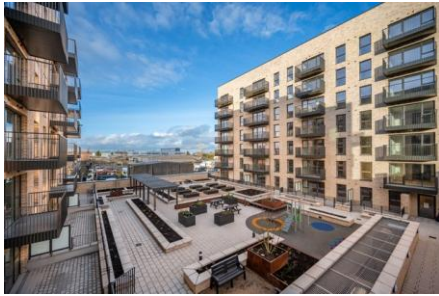
Innovation Square Apartments heated from the Heat Works District Heating Energy Centre located on the Belgard Road in Tallaght
